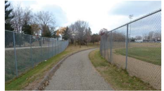
Drainage issues on Field 2.
