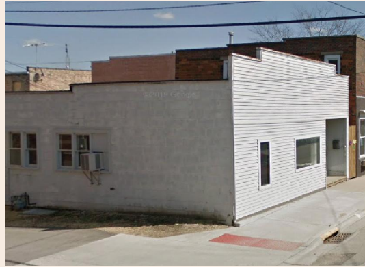
Before and after of a colorful conversion in Stockton, Illinois
